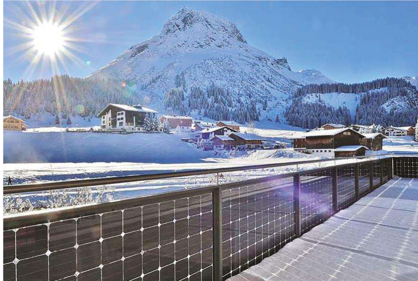
Fig. 9 BIPV balcony application [8].
