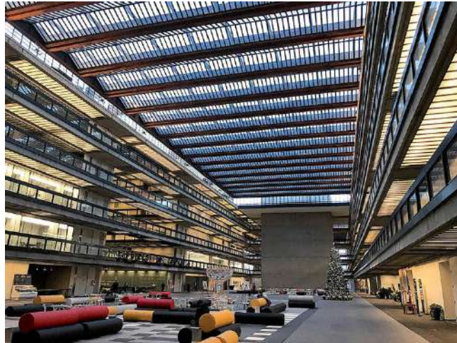
Fig. 3 PV skylight at Bell Works [5].
